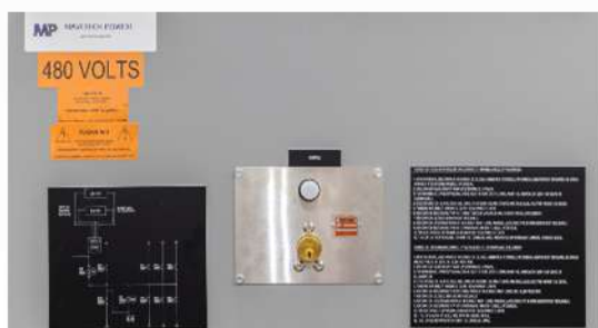
UPS Maintenance Bypass Switchboard with SKRU and Bypass Procedure
